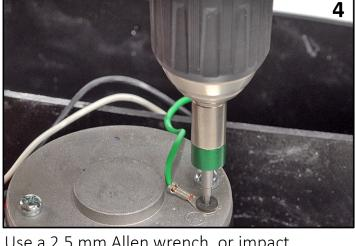
Use a 2.5 mm Allen wrench, or impact driver/drill, to remove the motor ground screw.
