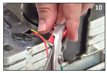
Clamp down using pliers. Repeat steps 9 and 10 with the black wire from the motor and the black wire from the harness.
