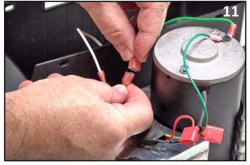
Connect the two white wires and the two black wires.
