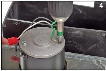
Use a 2.5 mm Allen wrench, or impact driver, to remove the motor ground screw.
